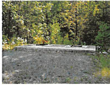
Figure 10: On Grade Slab September 2008
